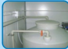
热熔焊接PP管路代替PVC
