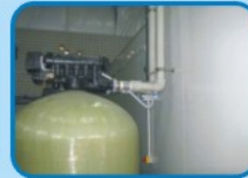
热熔焊接PP管路代替PVC
